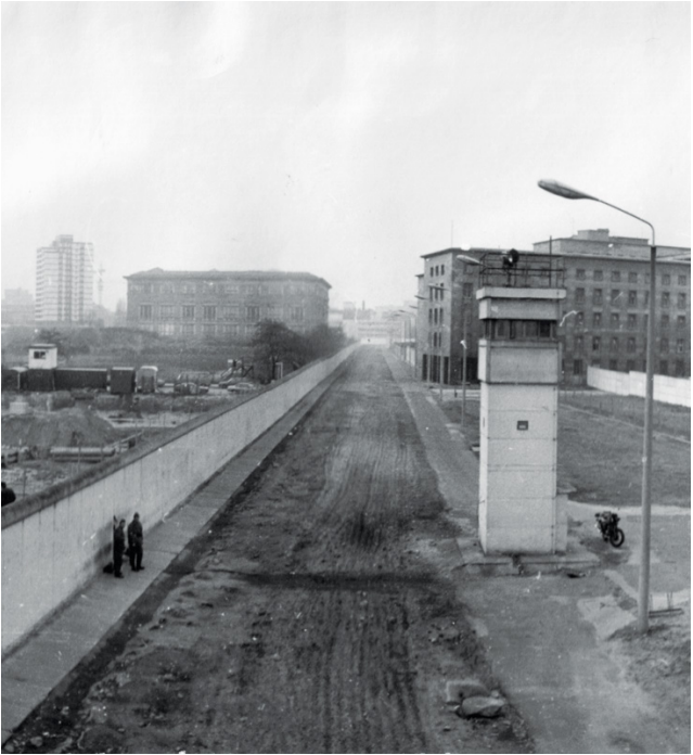
7 Gropiusbau and House of Ministries (now Federal Ministry of Finance), Berlin-Mitte, 1980s. < West / East >
