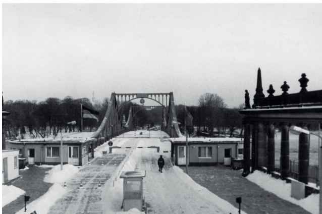
15 Glienicke Bridge, Potsdam, 1980s. Coming from Potsdam, East Germany, heading for West Berlin.
